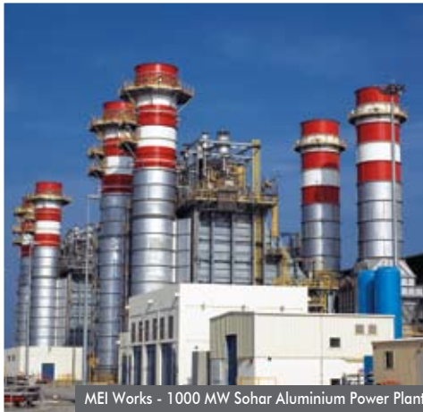
MEI Works - 1000 MW Sohar Aluminium Power Plant
