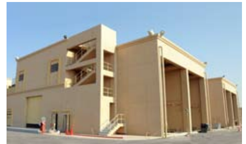
DubaiLand-2 Sub-station Project for DEWA/Siemens
