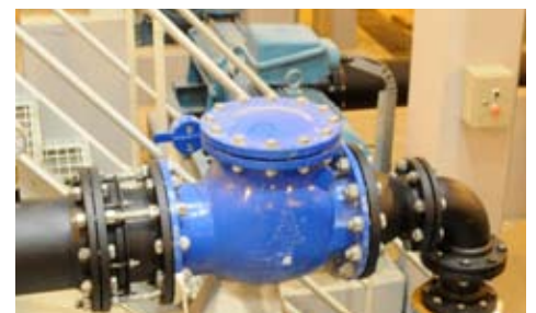
200+ Pumps supplied to 25 PAEW Projects
