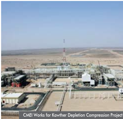
CMEI Works for Kawther Depletion Compression Project
