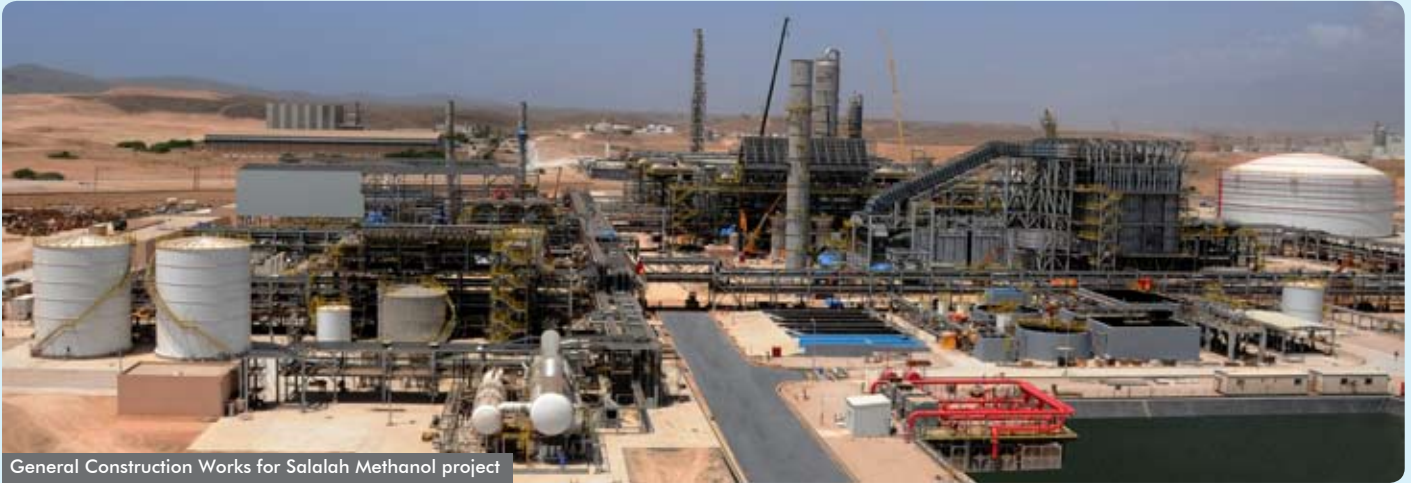
General Construction Works for Salah Methanol project
