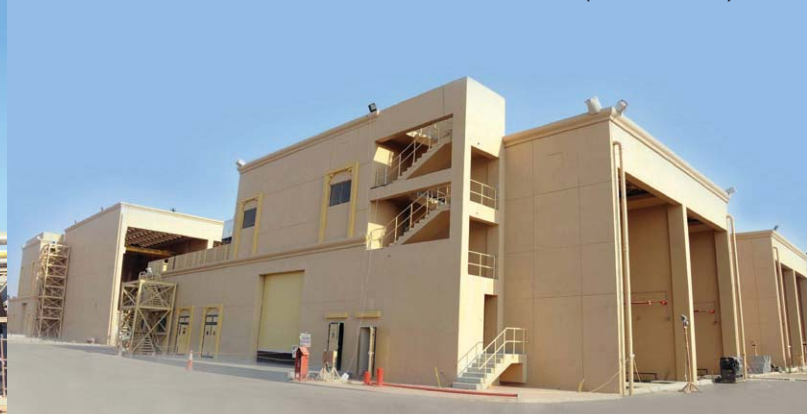
400/132 kV Dubailand-2 DEWA Sub-station (Civil Works)
