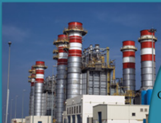
Sohar Aluminium Project - Oman's Largest Power Plant
