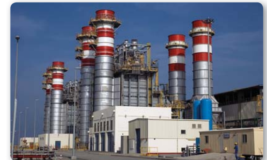
Sohar Aluminium Project
