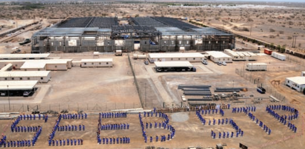
A' Seeb Sewage Treatment Plant
