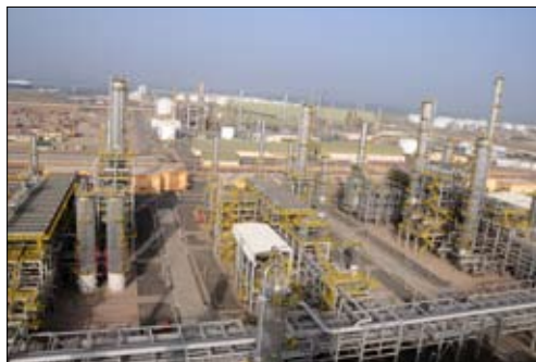
General Construction Works for Sohar Aromatics Projects.
